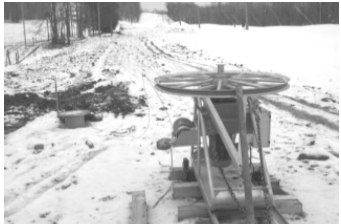
Figure 2 - The bottom of Hunt Hollow's new surface lift being installed.
